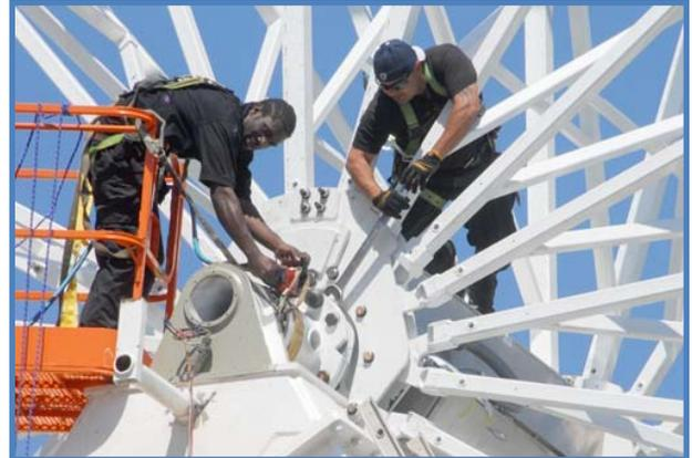
Figure 1 – Mechanics work at the axle as they assemble and maintain a huge Ferris Wheel.
